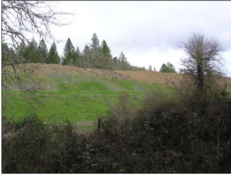
Observation 1 – Man-made berm with multiple burrows at MP 137.0.
