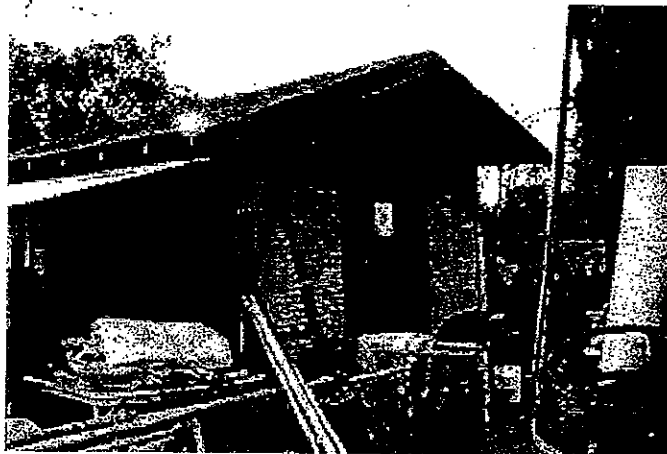
Shed (facing northwest)
