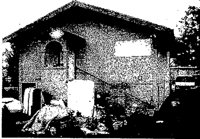
Rear of 1090 Jennings Ave. house
