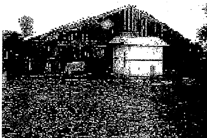
Barn facing east.
