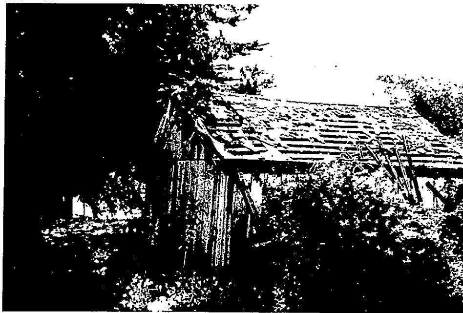
Garage, view toward northeast, roll 3, exposure 5 July 5, 1995
